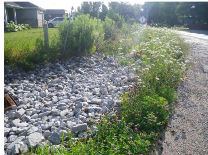
Image 20: View of large granular material around drainage catch basin (associated with the extant watermain).
