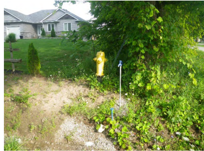
Image 10: View of disturbances associated with buried utilities (watermain).
