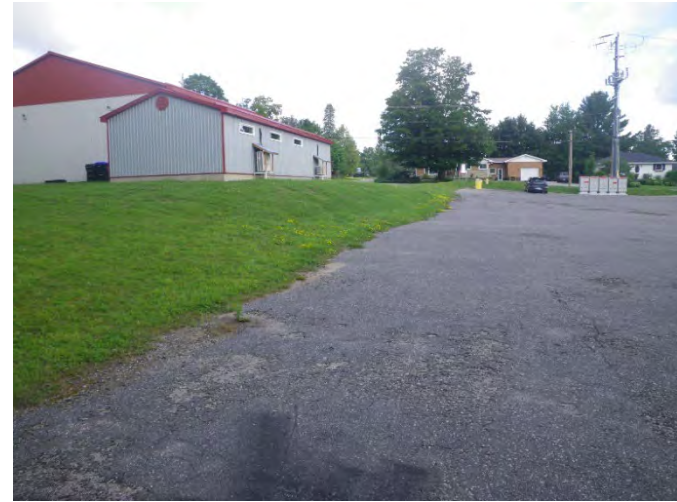
Image 18: View of disturbances associated with paved parking area.
