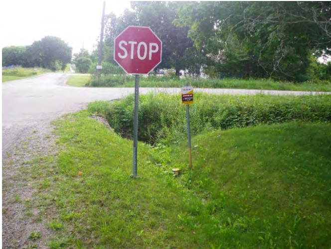
.Image 13: View of disturbances associated with buried utilities (gas main and gas service line).
