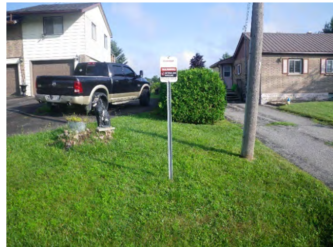
Image 12: View of disturbances associated with buried utilities (gas main and gas service line).
