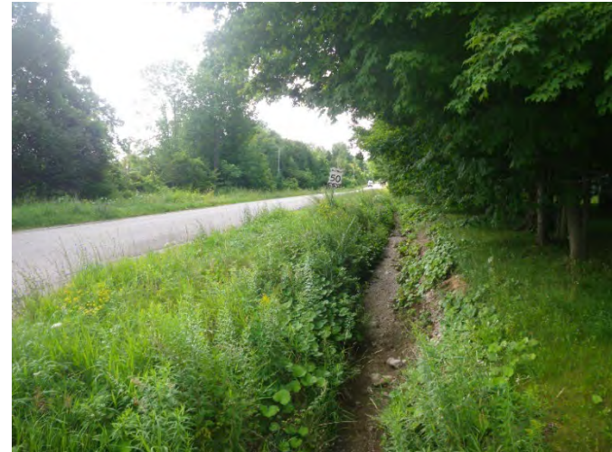
Image 6: View of disturbances associated with roadside ditching.
